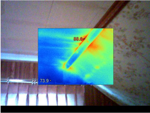
Photo # 1a Remove hardboard material and replace drywall
