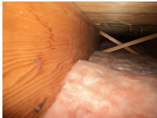
Photo # 3 Block & seal open attic crawl space floor with insulation stuffed into plastic bags and sealed with spray foam
