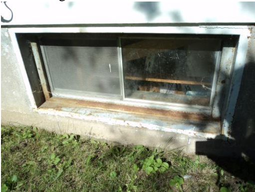
Photo # 7 Replace basement windows with insulated sliders or glass block & insert
