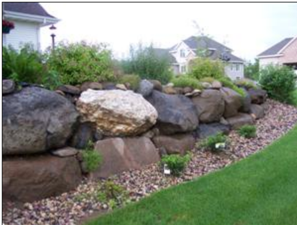
2.4 Picture 2 Retaining wall
