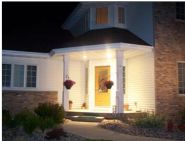
2.0 Picture 1 Front entrance
