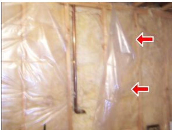
5.1 Picture 1 Basement wall & water pipe
